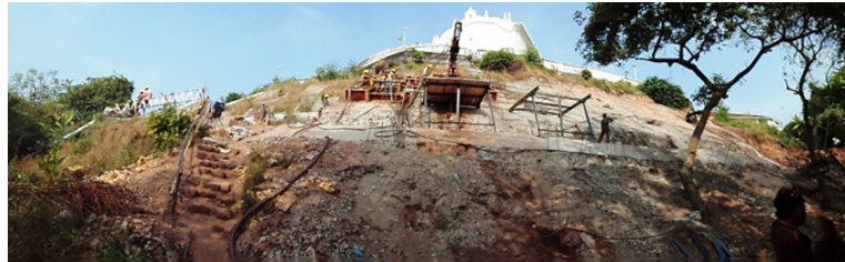
In-place inclinometers and piezometers installed for online slope monitoring at Cabo Fort, India
